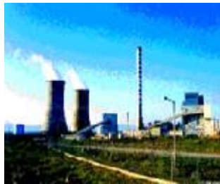
Electric Power Plant of Amynteon-Filota
